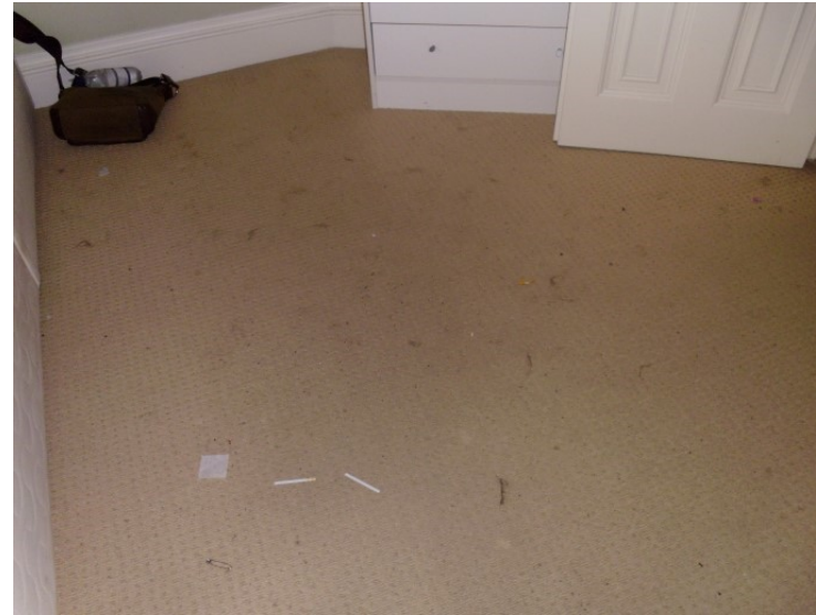
Bedroom – dirt and debris to carpet
